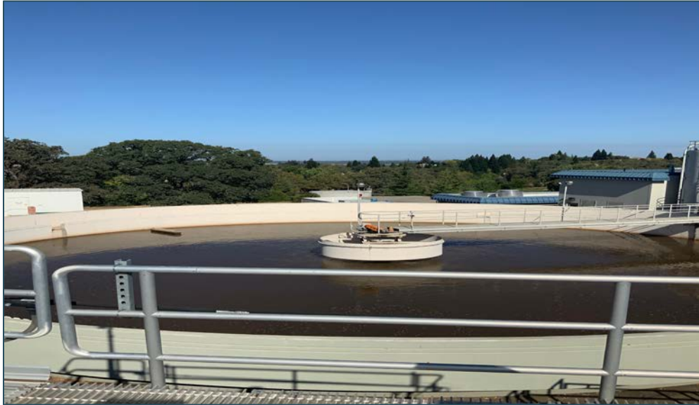
Figure 1-1: El Dorado Hills water treatment plant, secondary clarifier
