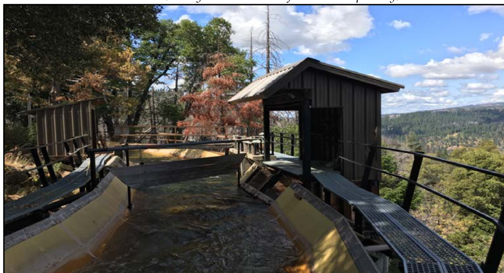
Flume 48 (a 60-year-old wooden flume with spillway)
